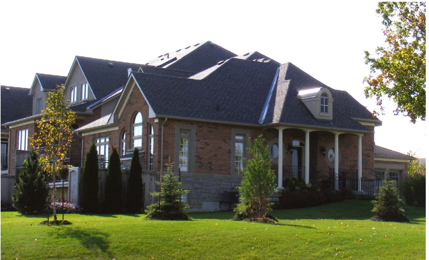
Figure 42 - Façades flanking/backing onto an open space should utilize a consistent level of architectural detail as front façades
