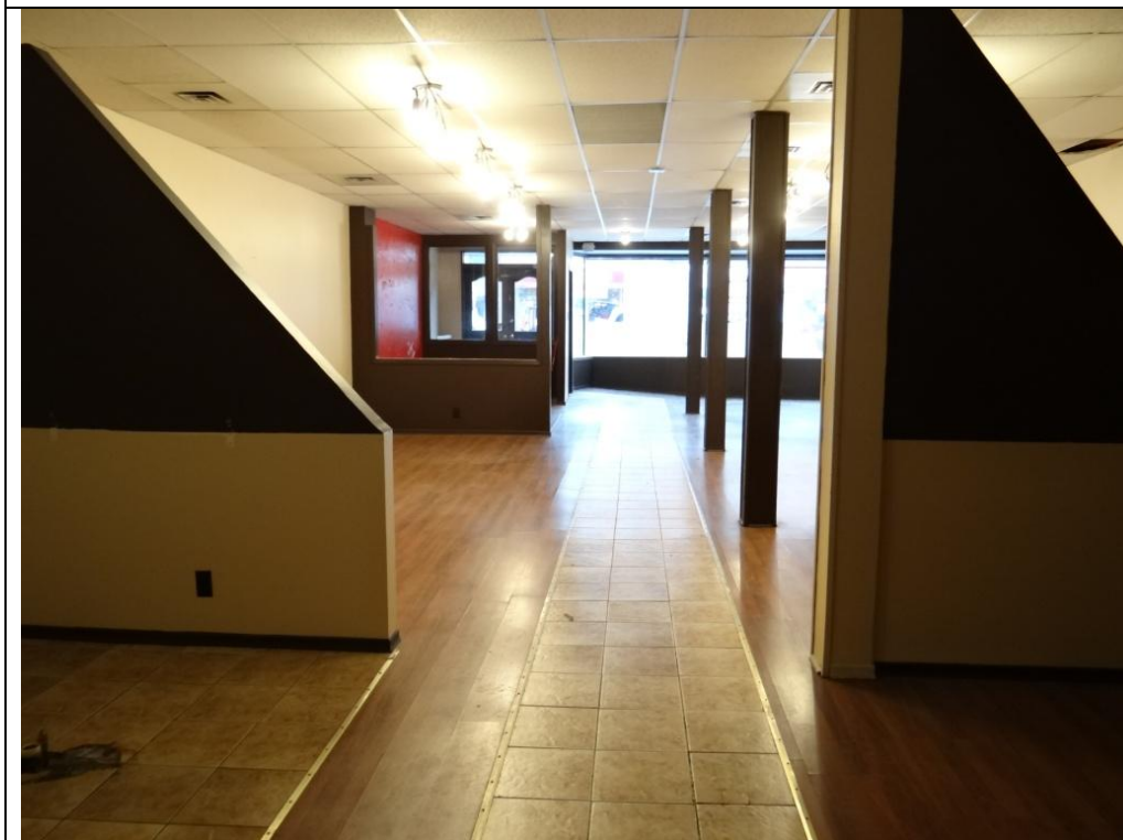
Plate 10: Interior of former salon at 69 Main Street South, looking west towards Main Street.
