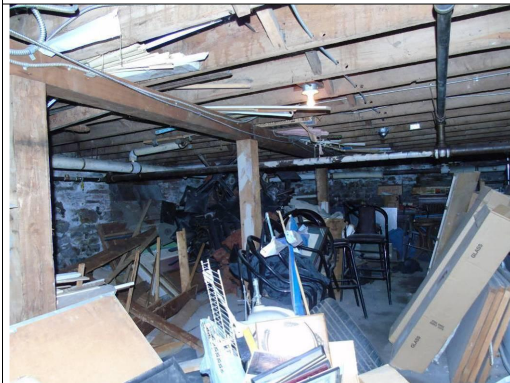
Plate 66: Basement of 71- 77 and 79 Main Street South, showing stone foundations, sawn beams, and modern dimensional lumber floor joists.
