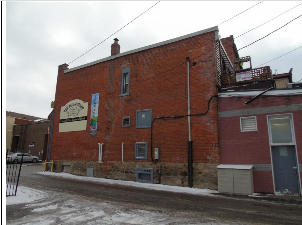
Plate 21: East elevation of the structure at 94-96 Mill Street, looking southwest.
