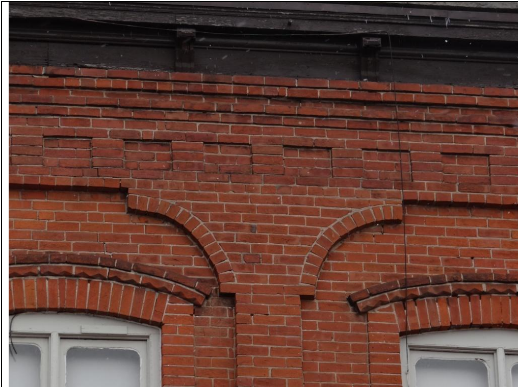
Plate 43: West elevation of 79 Main Street South, showing decorative brickwork, roof bracketing and segmental arches on the window, looking east.
