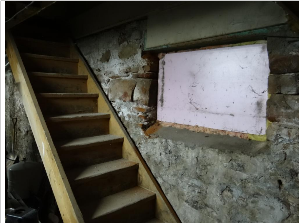
Plate 29: Detail of foundations, blocked windows, and un-used stairs in the basement at 94-96 Mill Street.
