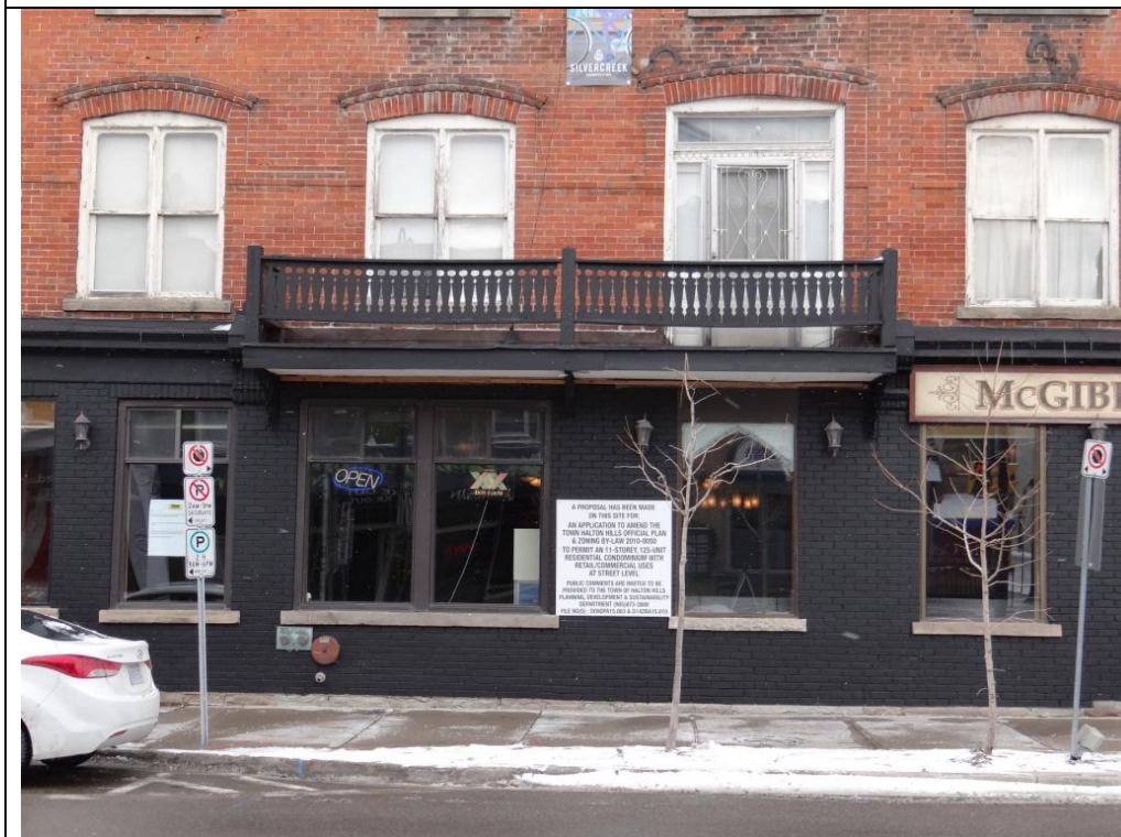
Plate 46: West elevation of 79 Main Street South, showing ground level windows and brickwork, looking east.
