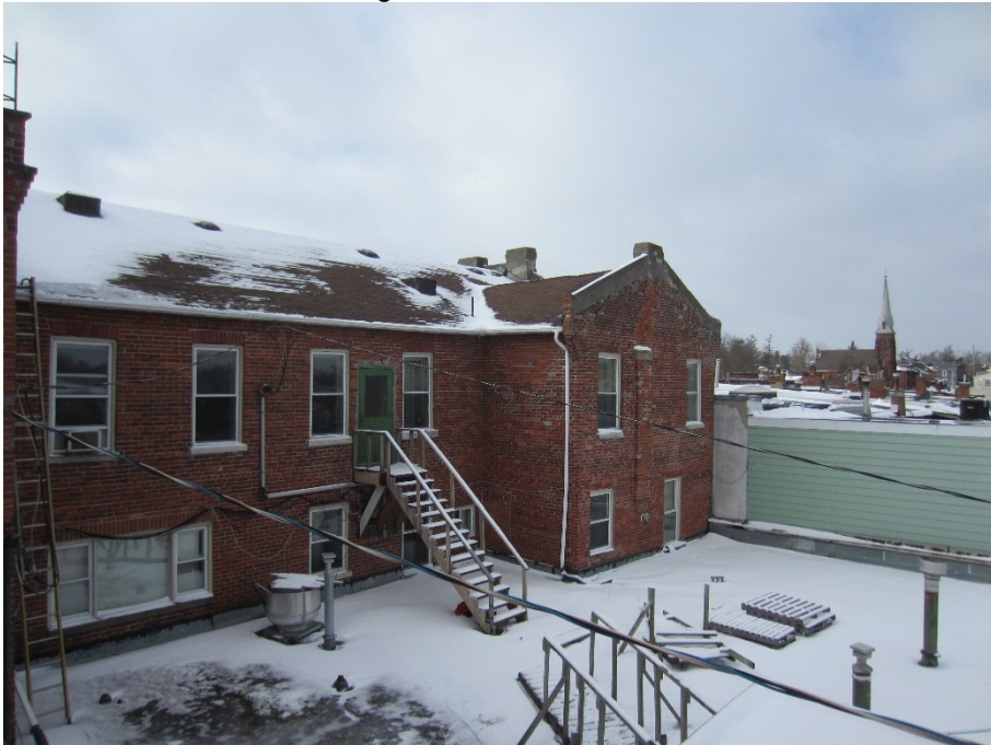
Photo #6: Side of the building
