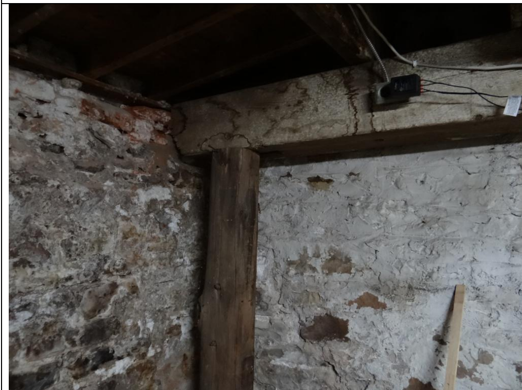
Plate 30: Detail of the foundation and large support beams in the basement at 94-96 Mill Street.
