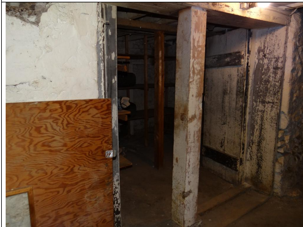
Plate 14: Wooden support posts in the basement of 69 Main Street South.
