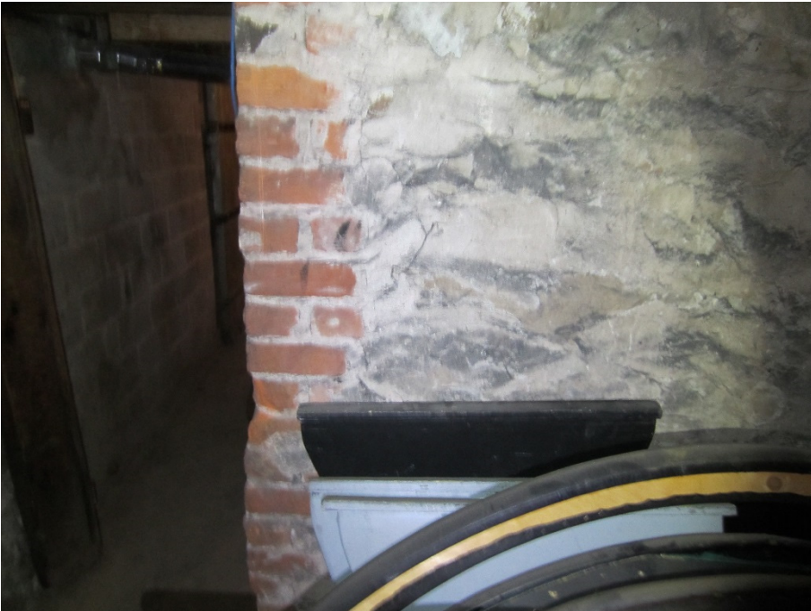
Photo #12: Basement brick foundation
