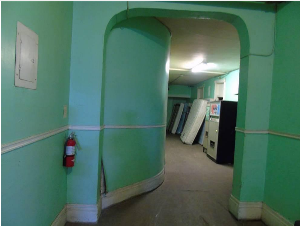
Plate 56: View of the main hallway on the second floor, looking east. Note that the hallway jogs to the south.
