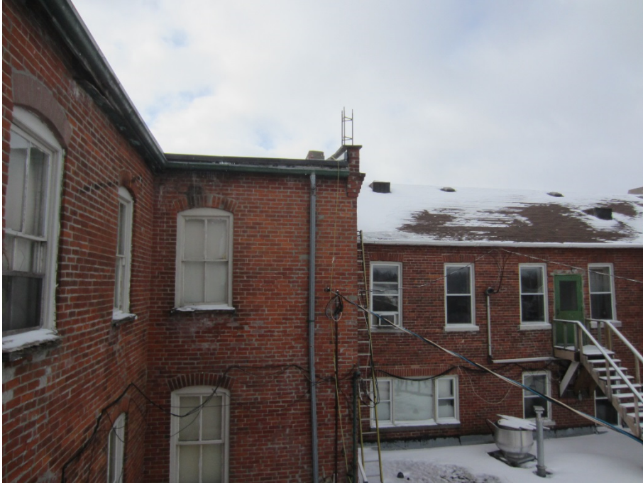
Photo #5: Side of the building
