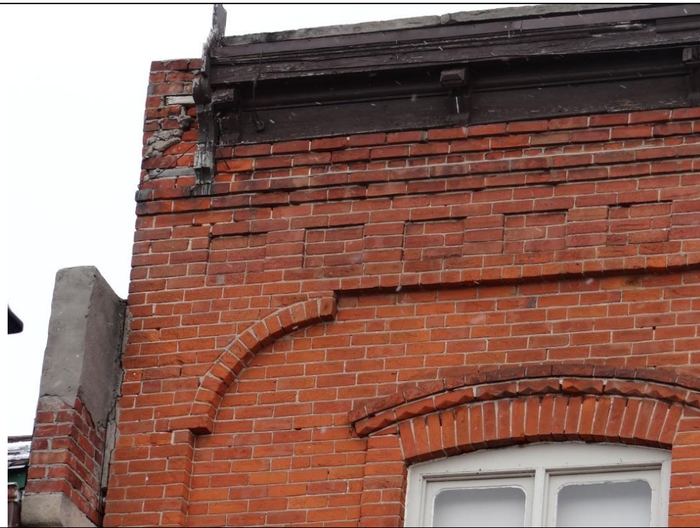
Plate 42: West elevation of 79 Main Street South, showing decorative brickwork, roof bracketing and segmental arches on the window, looking east.
