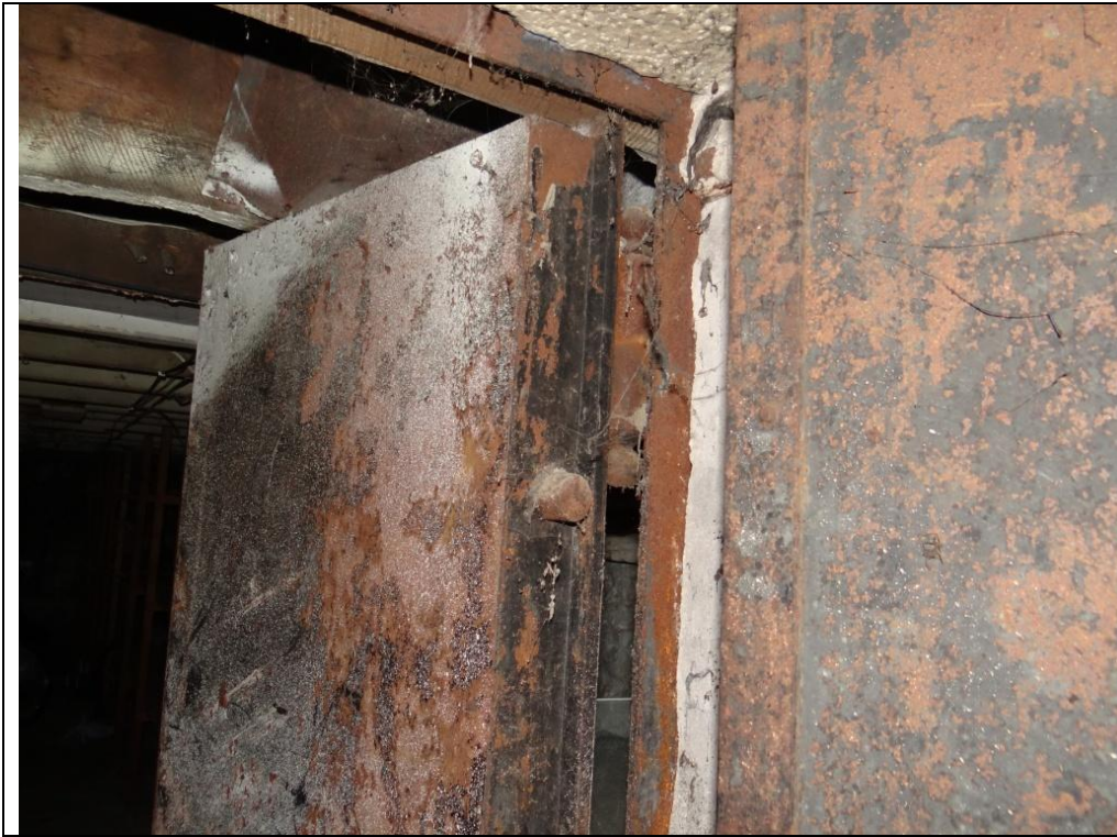
Plate 15: Detail of the Bank of Hamilton vault door in the basement of 69 Main Street South.
