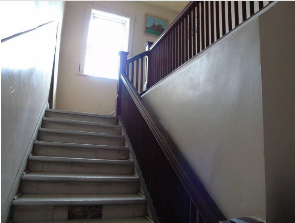
Plate 60: Staircase leading from the restaurant up to the second floor.
