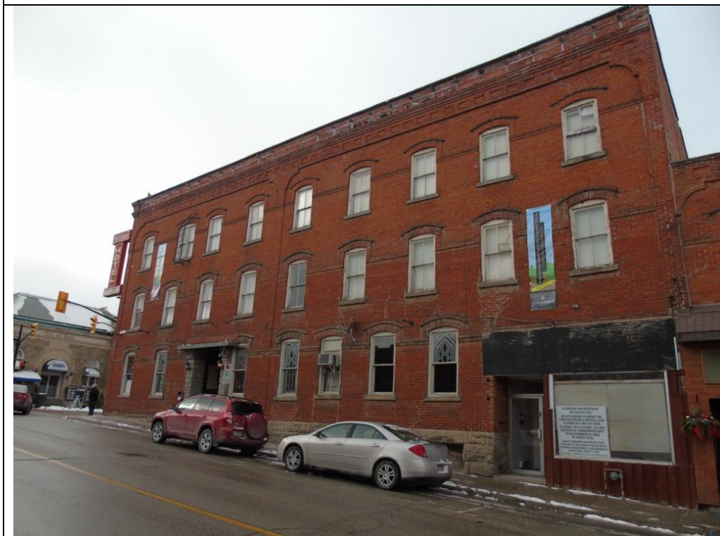
Plate 48: South elevation of 79 Main Street South, looking northwest.
