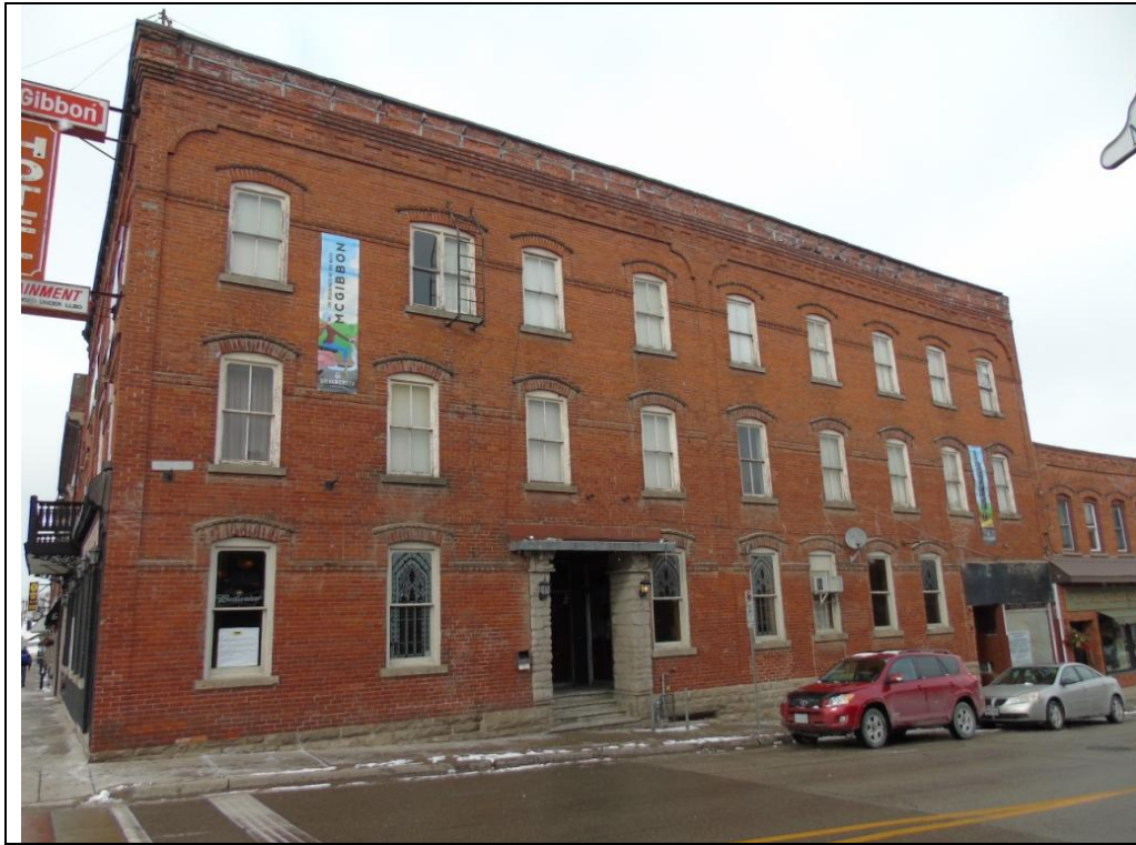
Plate 47: South elevation of 79 Main Street South, looking northeast.
