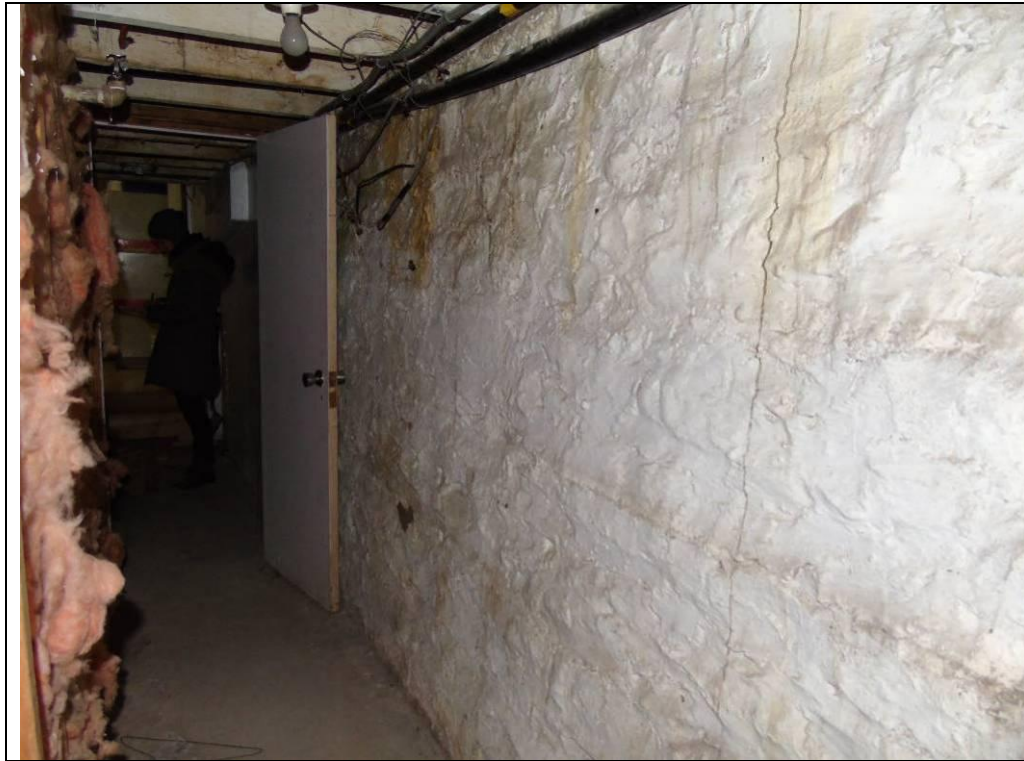
Plate 69: Basement of 71- 77 and 79 Main Street South, showing painted stone foundations at right, and modern insulated walls at left.
