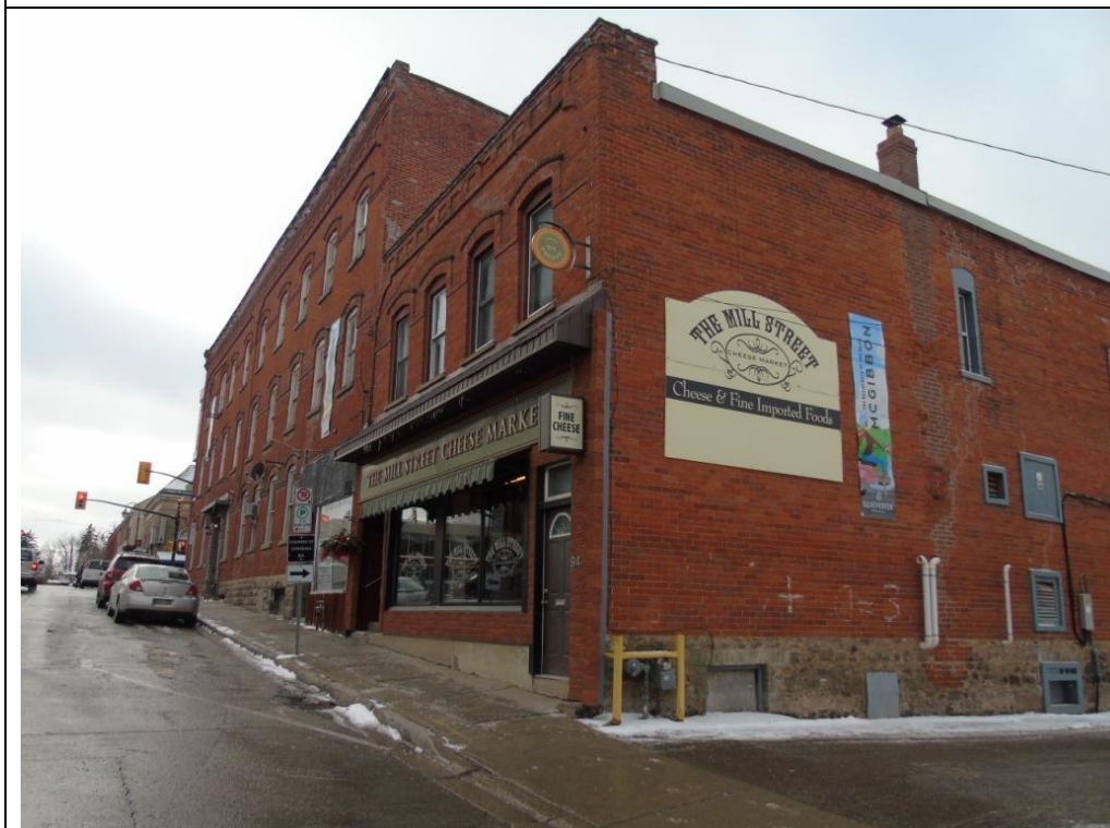
Plate 20: South and east elevations of the structure at 94-96 Mill Street, looking northwest.
