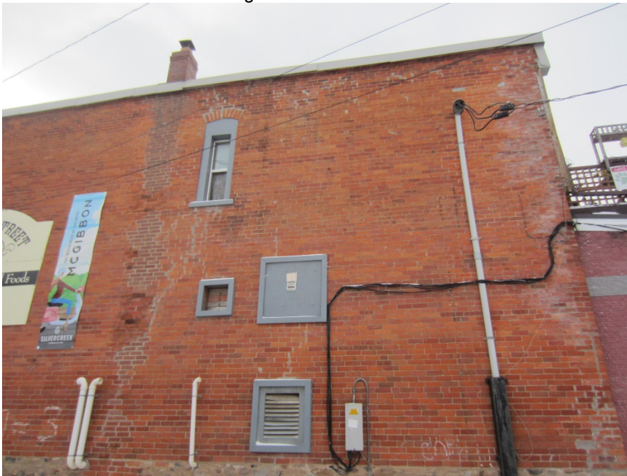
Photo #4: Back of the building
