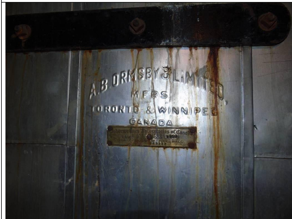
Plate 72: Basement of 71- 77 and 79 Main Street South, showing heavy metal boiler room door.
