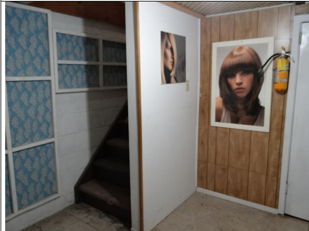
Plate 16: Detail of the finished section of the basement in the concrete block addition at 69 Main Street South.
