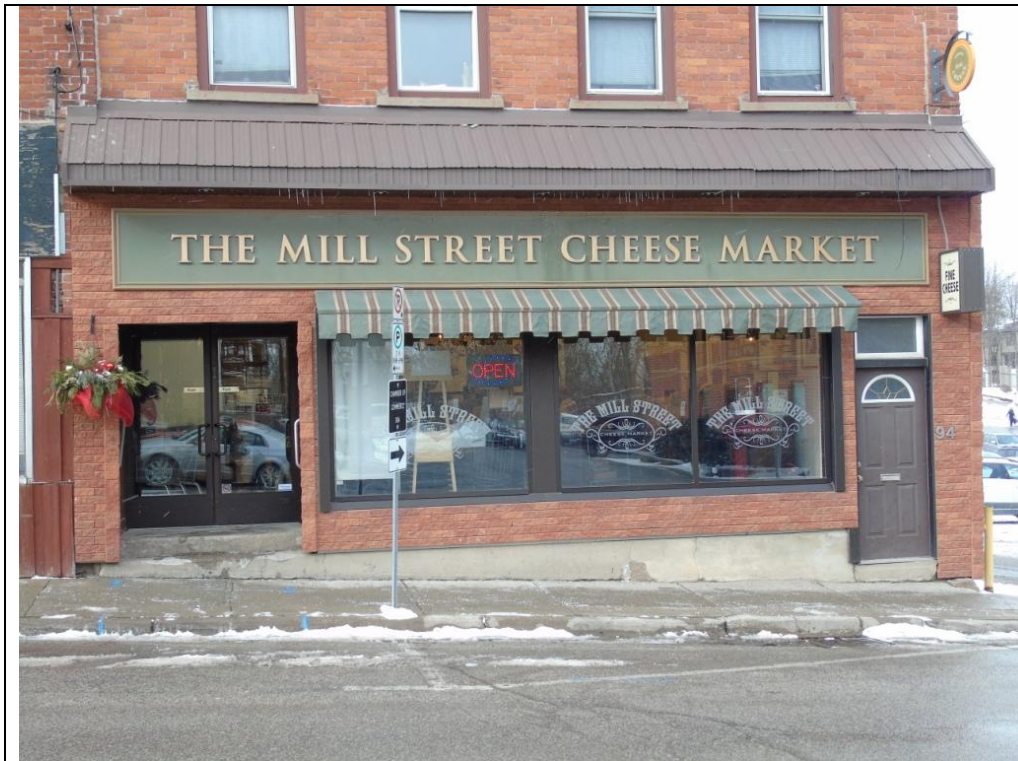
Plate 19: Detail of the brick work and large windows on the first floor of the south elevation of the structure at 94-96 Mill Street, looking north.
