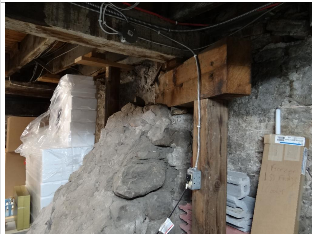
Plate 28: Detail of the stone buttressing and large support beams on the north wall of the basement at 94-96 Mill Street, looking northwest.
