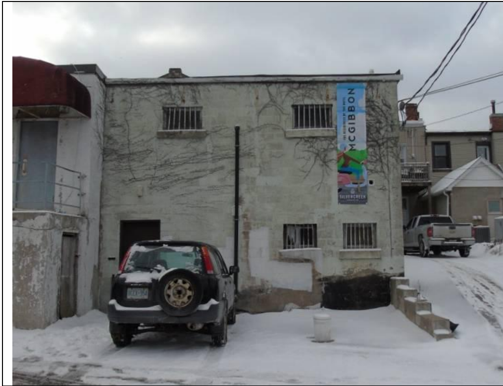
Plate 7: East elevation of the concrete block addition at 69 Main Street South, looking west.
