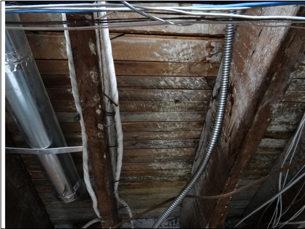
Plate 27: Detail of the sawn floor joists and softwood floor boards from the basement at 94-96 Mill Street.
