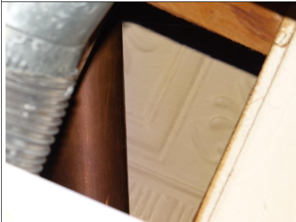
Plate 8: Detail of stamped tin ceiling tiles on original main floor ceiling of 69 Main Street South.
