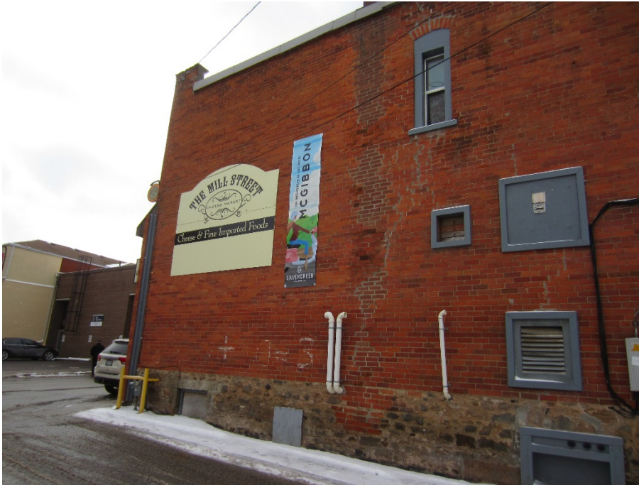
Photo #3: Back of the building
