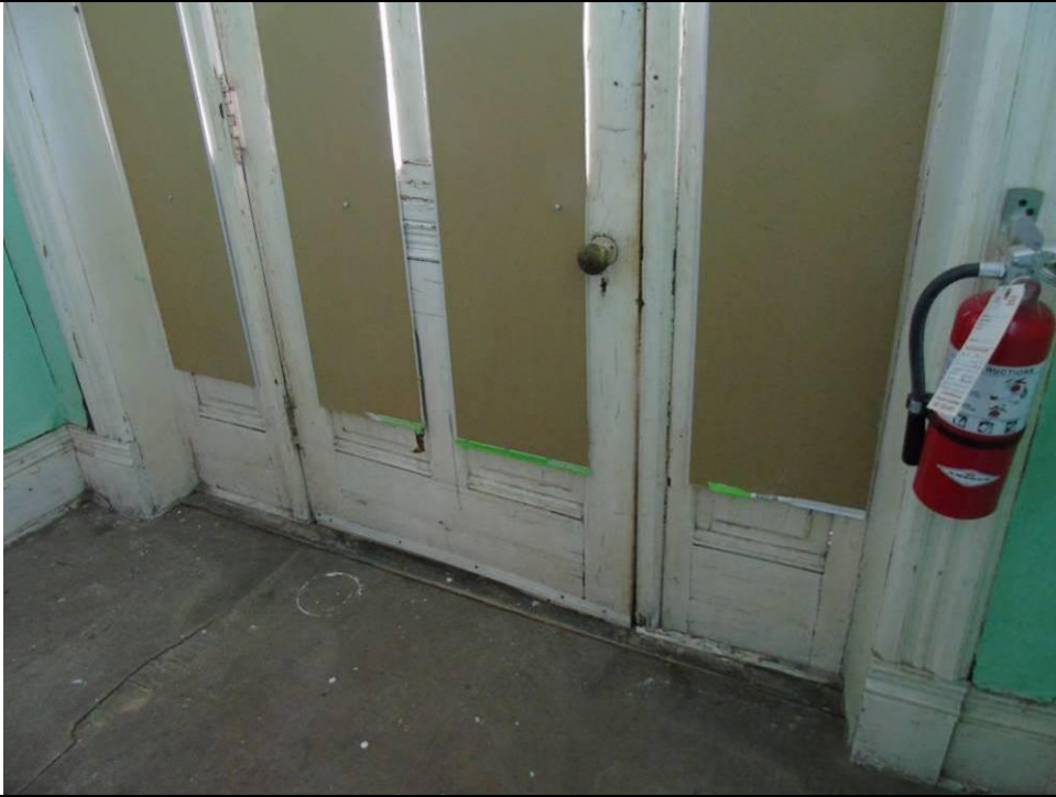
Plate 55: Detail of the original wooden door that leads out to the balcony on Main Street South.
