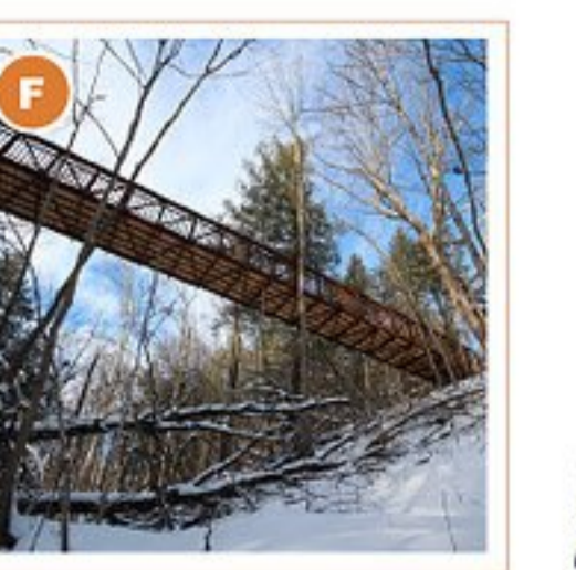
Regan Ridge Bridge
