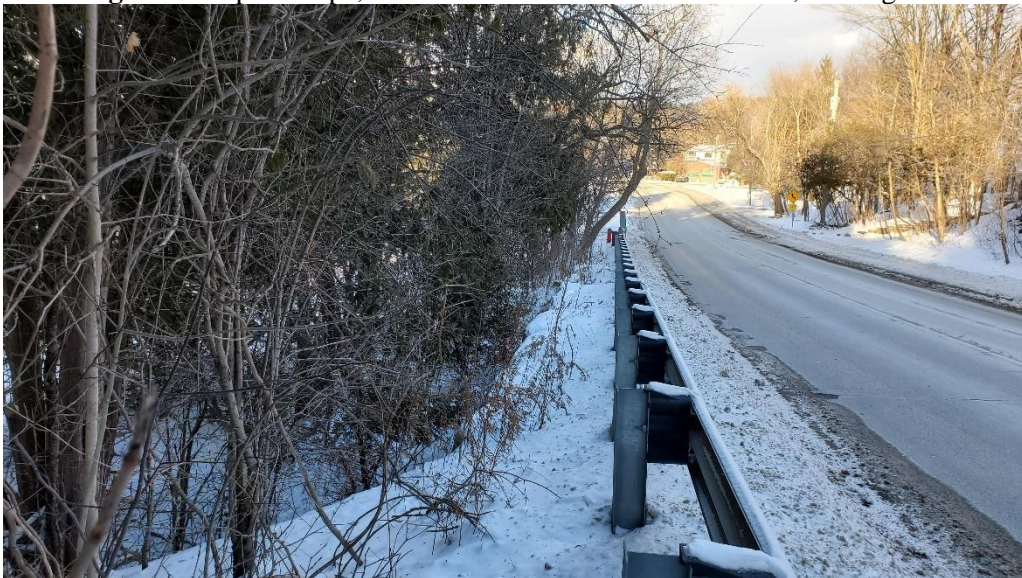
Figure 4: Top of Slope, between 27 and 33 Wildwood Road, looking east
