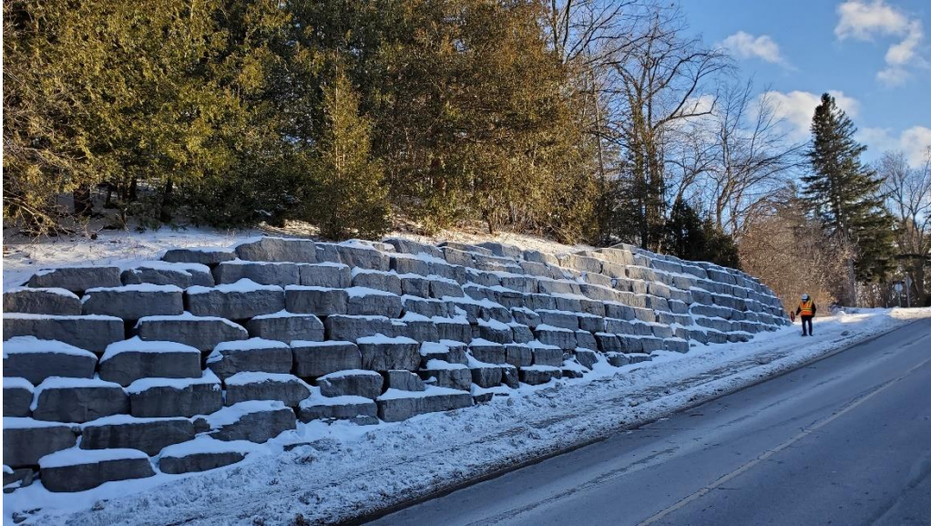
Figure 1: Armourstone retaining wall, south of street, 33 Wildwood Road
