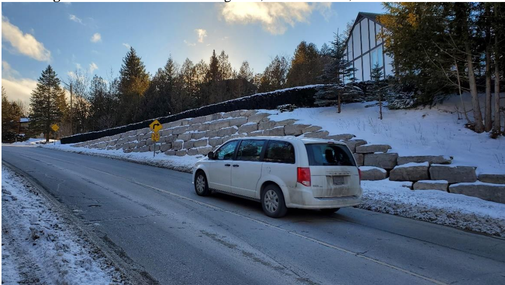
Figure 2: Armourstone retaining wall, north of street, 33 Wildwood Road
