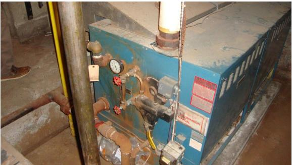
Photo 8: View of the gas fired furnace within basement; utilize for heating 79 Main Street South building
