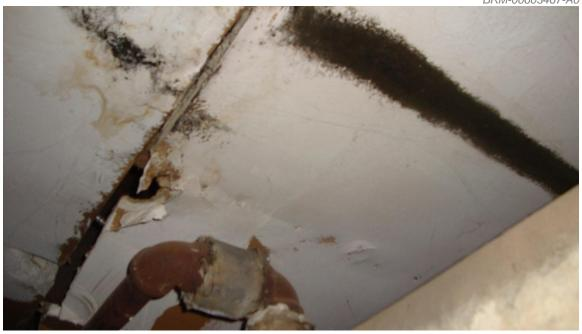
Photo 13: View of mould on ceiling -79 Main Street S building
