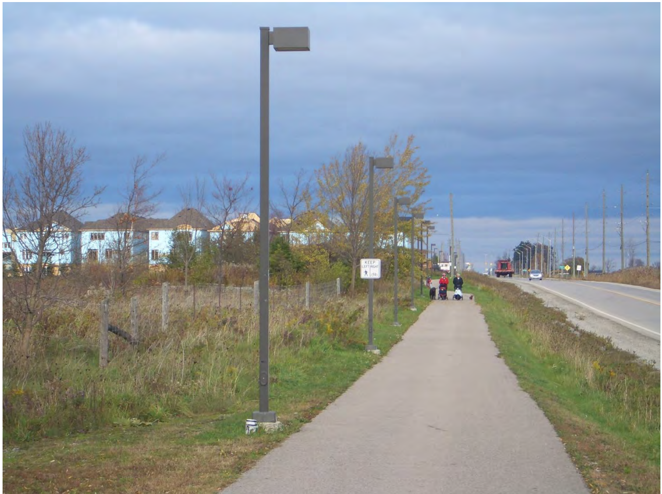
Light-emitting diode (LED) lights along 10 th Side Road demonstrate the use of innovative lighting technology while reducing energy use.
