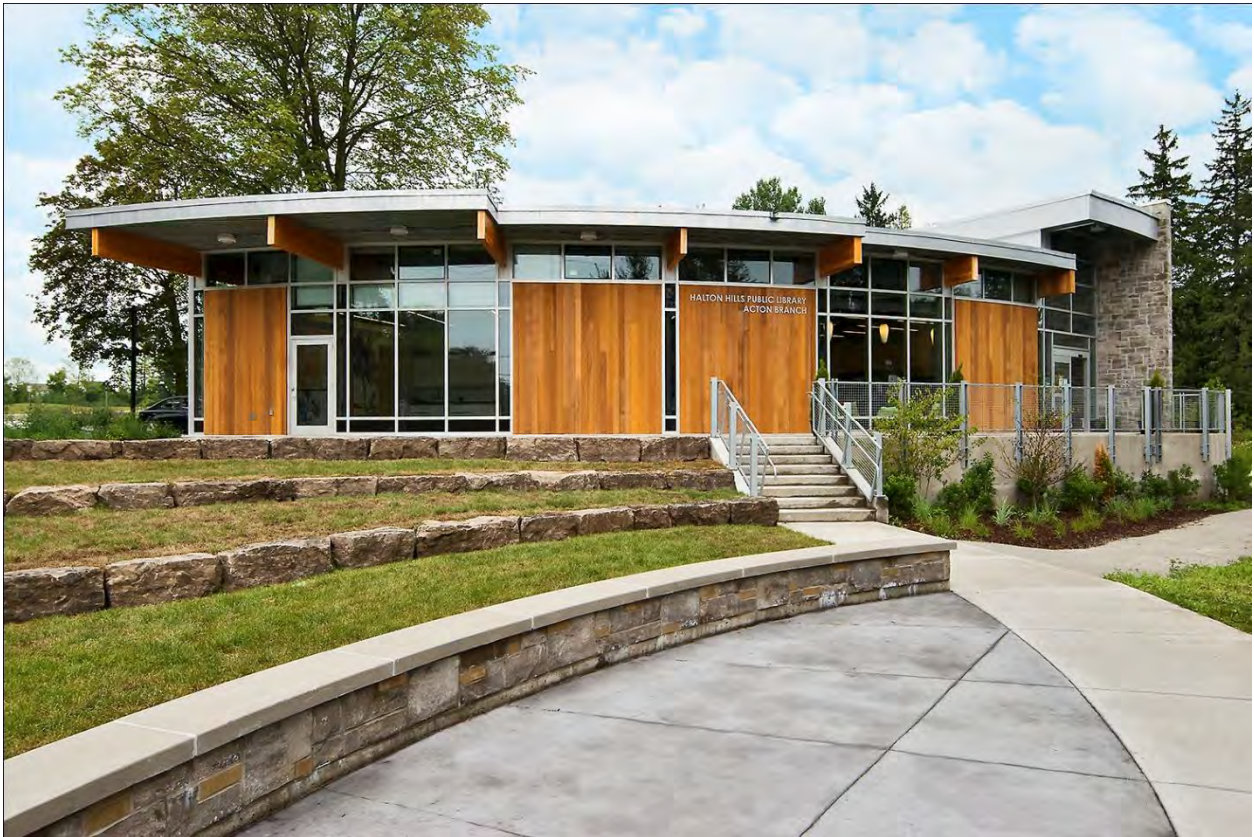
The Acton Branch Library is now LEED® Gold Certified, making it the Town's greenest facility!
