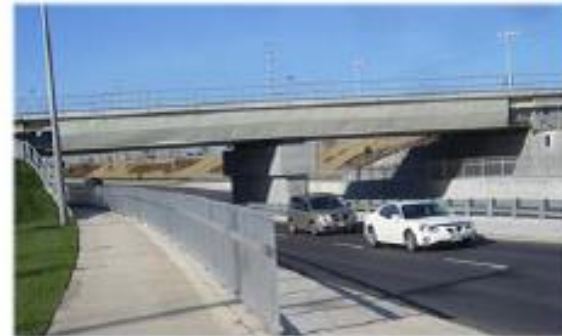
Example of Underpass Crossing
