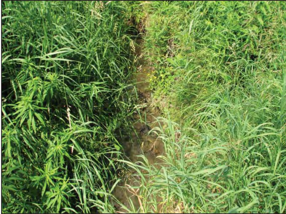
Highway drain 8 on 21 June 2007 (looking upstream); water in the channel due to groundwater discharge from Steeles Avenue construction activities.
