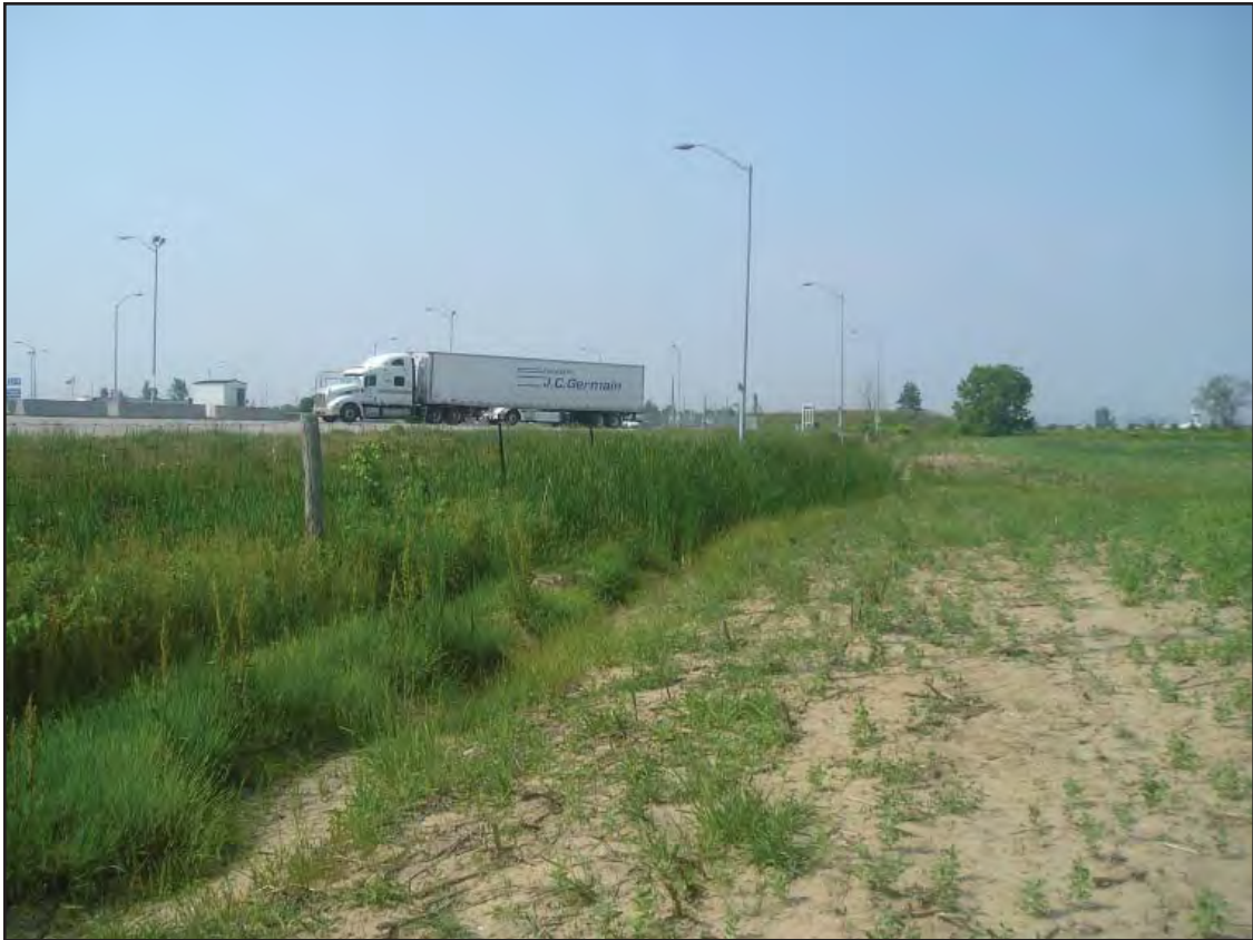
Highway drain 6 (looking downstream).
