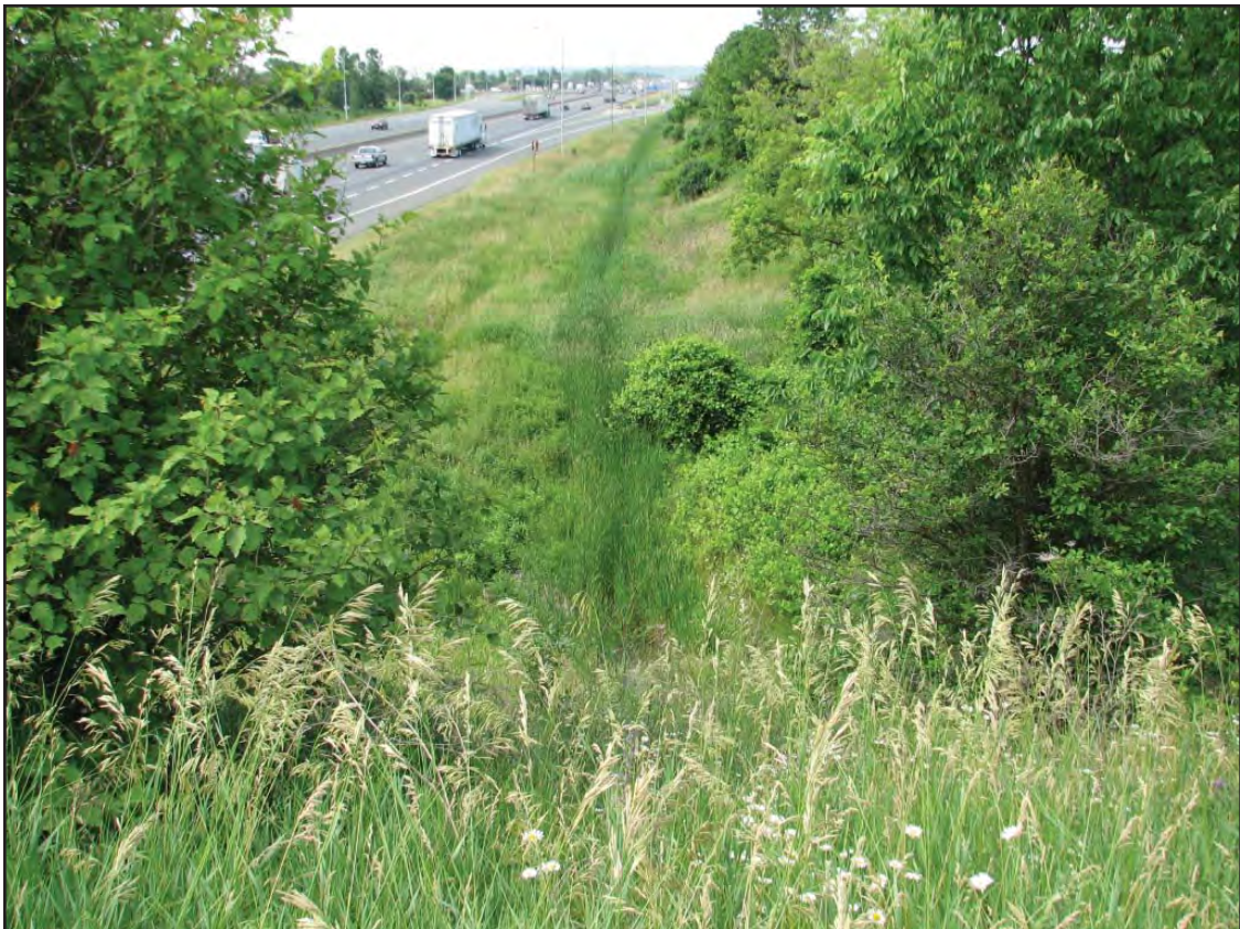
Highway drain 7 (looking upstream).
