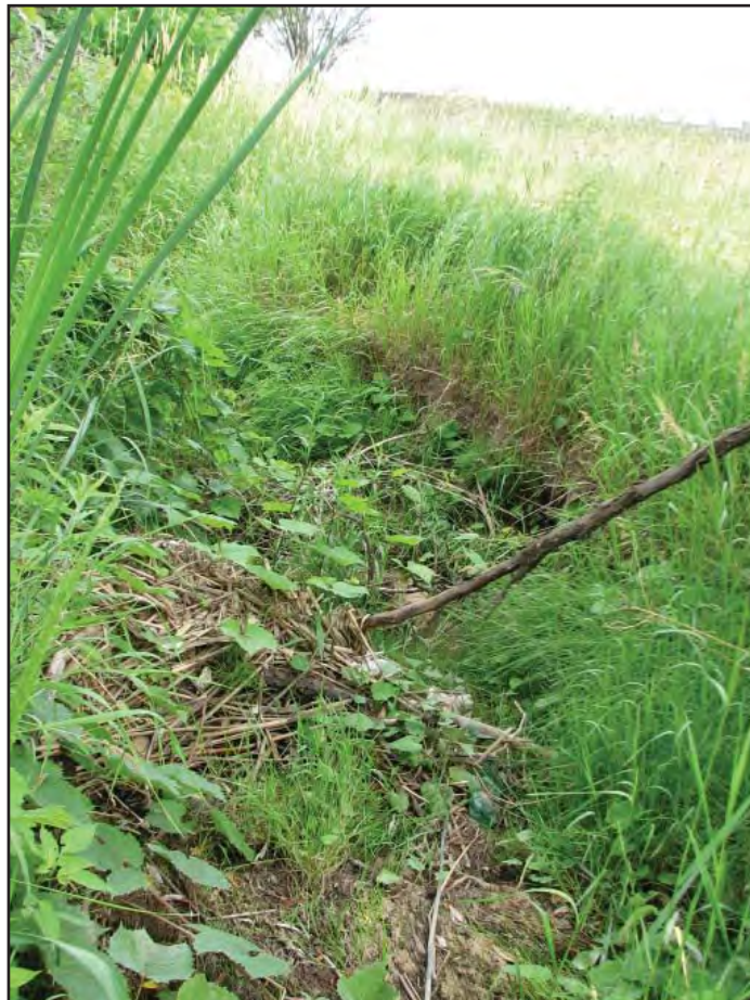
Highway drain 8 on 28 June 2007 (looking downstream).
