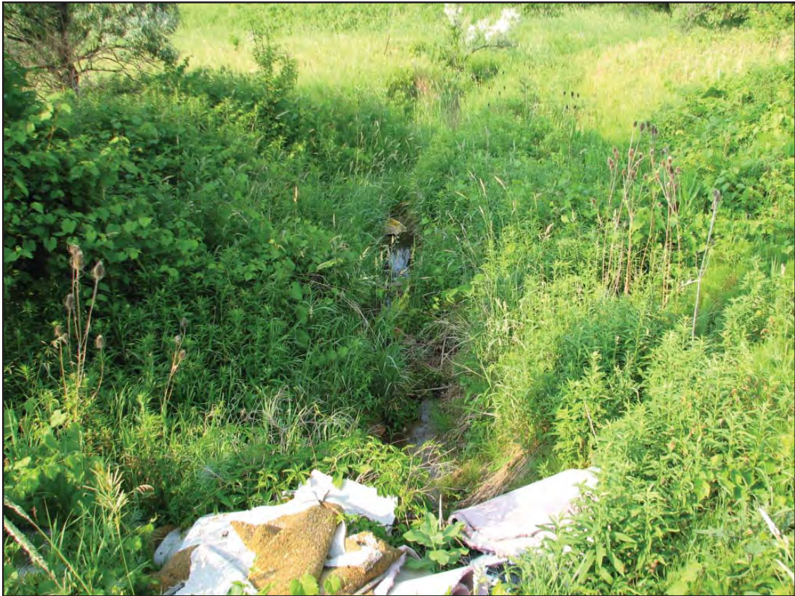
Highway drain 12 (looking downstream).
