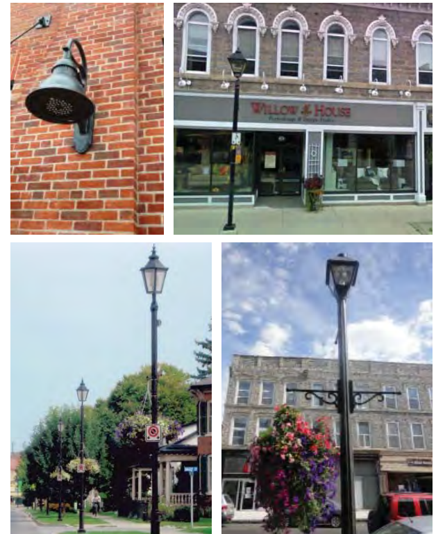
Above: Appropriately designed lighting fixtures add to the facade's aesthetic while offering nighttime visibility. Below: Light standards throughout Norval should reflect the historic character of the community.
