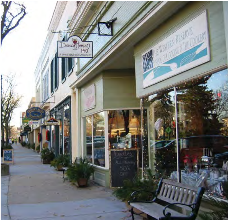
Buildings should be of uniform height to create a defined street ceiling.
