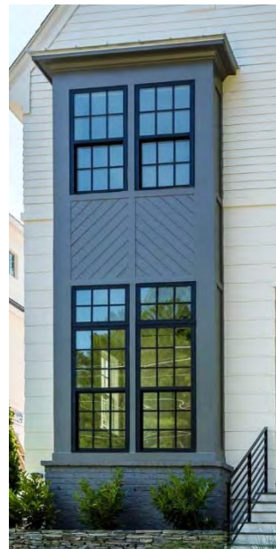
An example of a boxed-out window and grill pattern illustrating a continuous grill pattern and proportions from first to second floor
