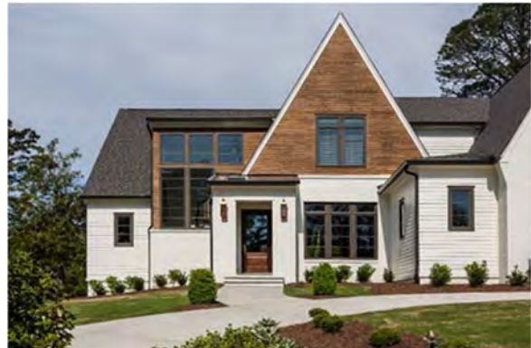
An example of contrasting wood siding in a white and stain grade with tone on tone brick work
