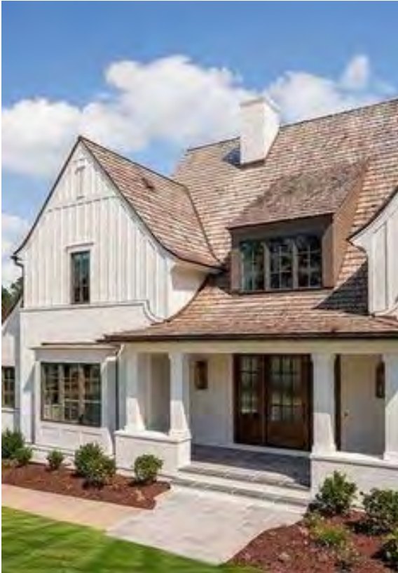
An example of porch columns, gable soffit trim, bay window paneling reflecting simple clean lines without overly accentuated moldings
