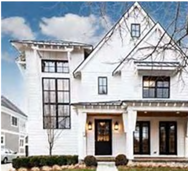
An example of a front covered porch, deep soffit overhangs and shallow gable overhangs
