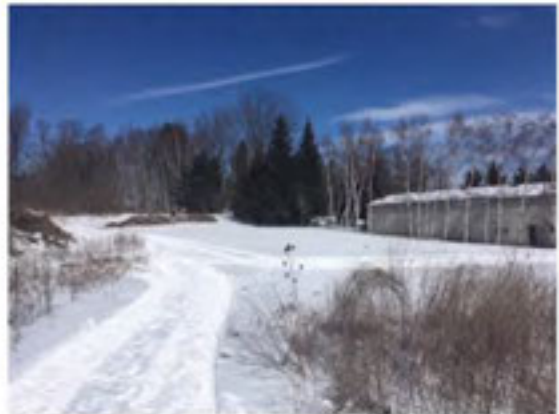
Picture 16: View of the east adjacent residential buildings, facing northeast.
