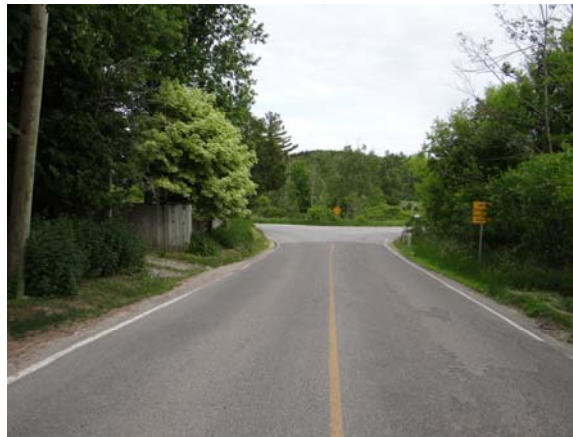
Churchill Road; south approach
