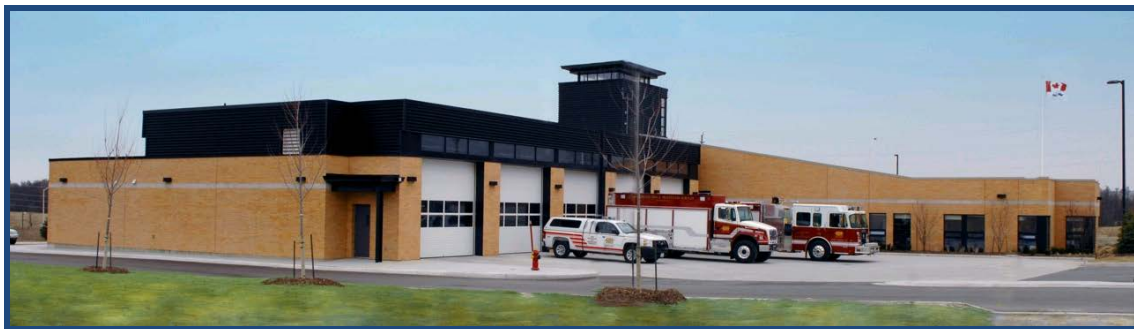
Figure 11 3: District 3 Station – Headquarters, Georgetown
