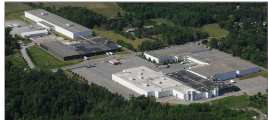
Saputo Dairy Processing Facility, 279 Guelph St., Georgetown Industrial Area.
