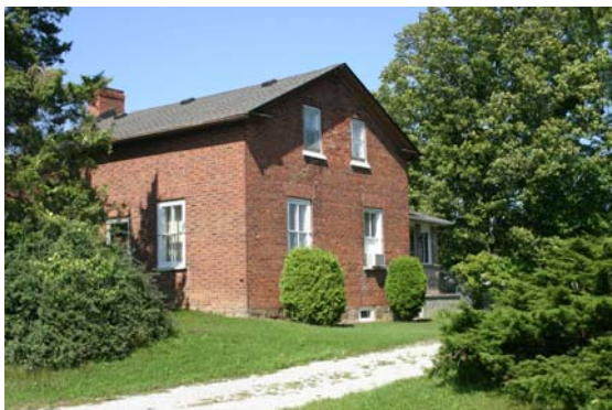
Plate 11: View of one of the houses fronting Trafalgar on Lot 14.
