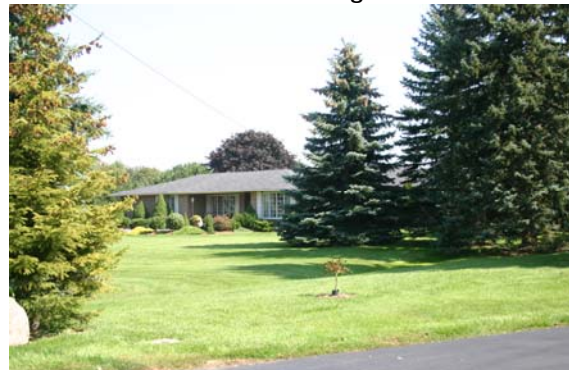
Plate 18: View of one of the houses fronting 15 Sideroad on Lot 15.
