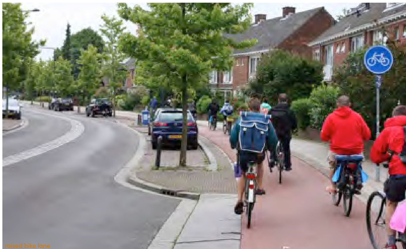
raised bike lane
