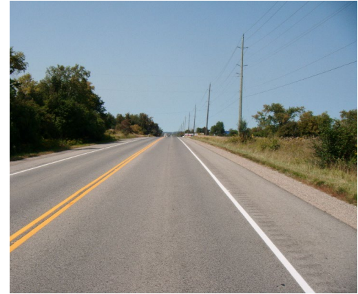
Rural Setting Partially paved shoulder
