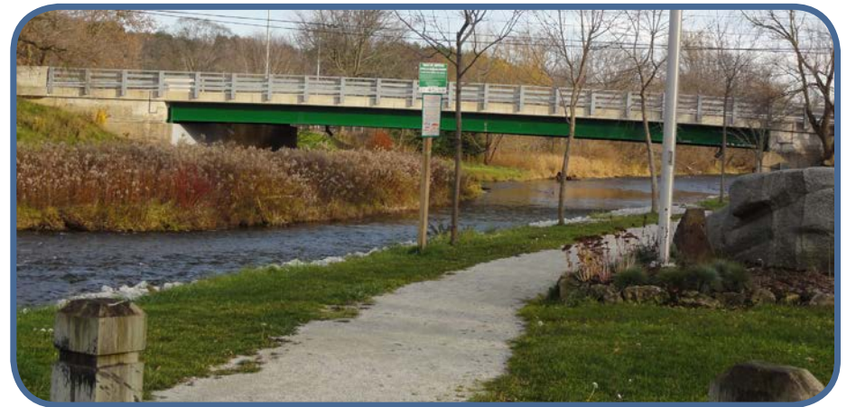
Glen Williams - Wildwood Road / Confederation Street
