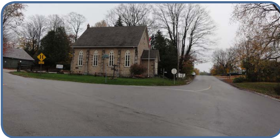
Limehouse - Fifth Line / Sideroad 22
