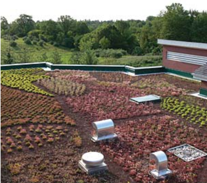
If a green roof is not accessible, maintaining native, low-maintenance plant species should be encouraged.
