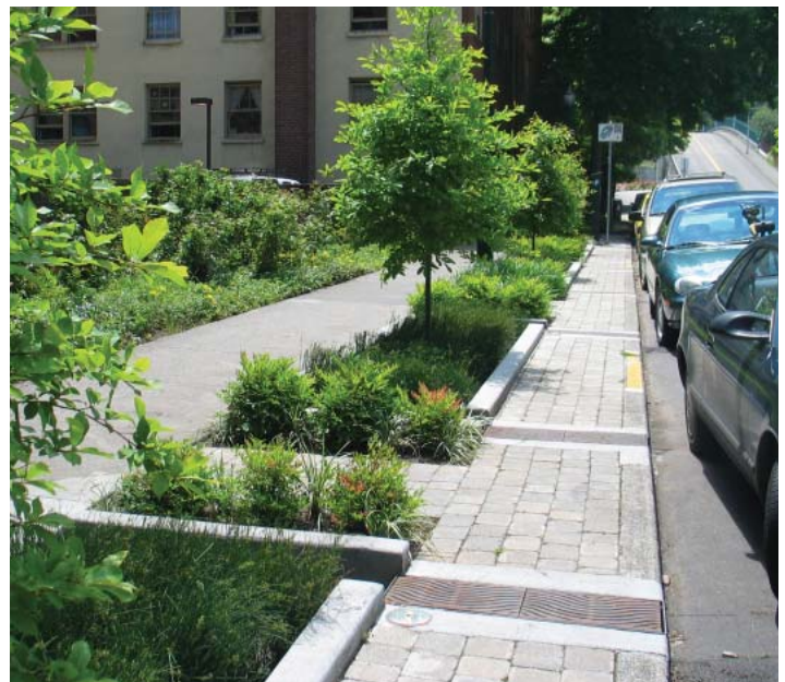
Landscaping with planters can manage stormwater run-off by directing water flows into planted areas.
