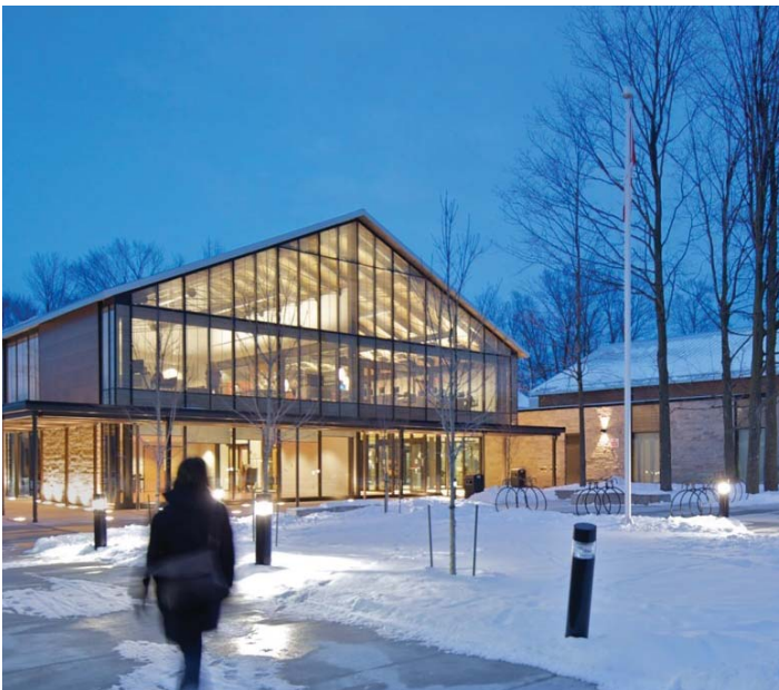
Community centres should incorporate high quality, durable materials, such as curtain walls.
