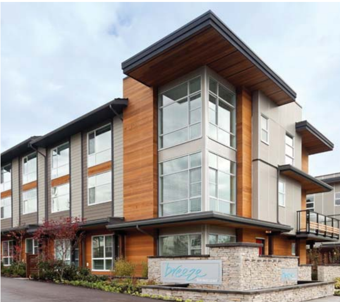
Wide roof overhangs are encouraged to provide shade and weather protection.
