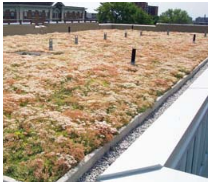
Green roofs are encouraged to achieve a minimum of 80% coverage of the total open roof space.
