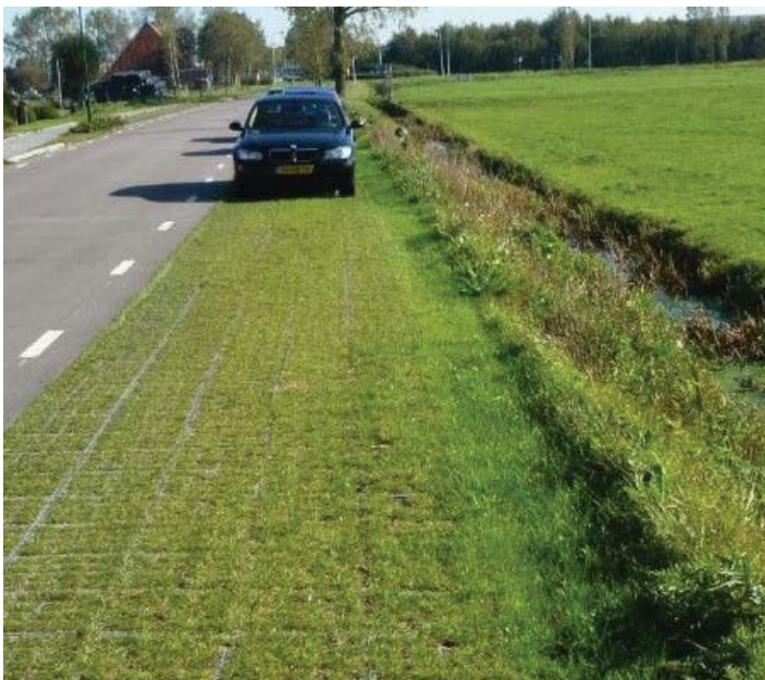
Semi-permeable paving techniques can help reduce water run-off and encourage ground water infiltration.
