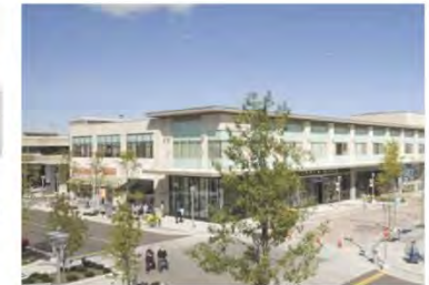
Large-format commercial buildings should be broken down into an appearance of multiple smaller buildings, through the use of vertical and horizontal articulation elements, recesses, projections and changes in material.
