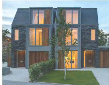
Both halves of semi-detached dwellings should be compatible in terms of design expression. They may be symmetrical or asymmetrical.
