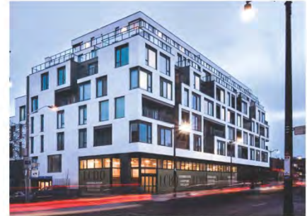
Mid-rise buildings should transition in height and massing, through the use of setbacks and recesses.
