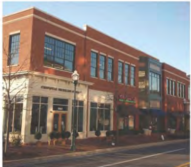
Ground floor commercial uses should incorporate prominent display windows adjacent to building entrances.
