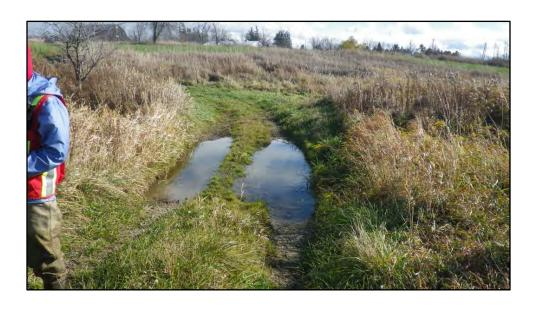
79. HT-2b-1 Farm crossing of channel with no CSP to convey flow.
