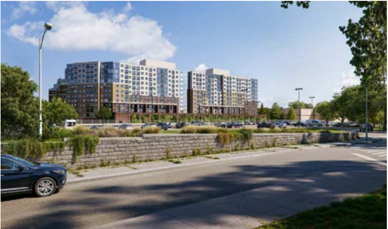
Figure 3-2: View of Buildings 1 & 2 from King Street taken at street level, Prepared by ICON Architects
