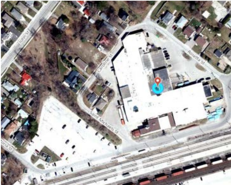
Figure 1. Aerial view of 1 Rosetta St, Georgetown, ON L7G 3P1
