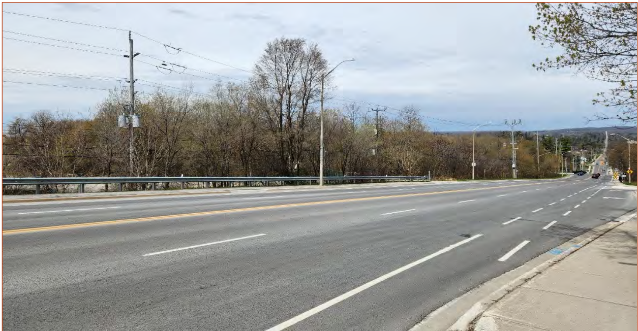
Image 1. View north on Mountainview Road North
