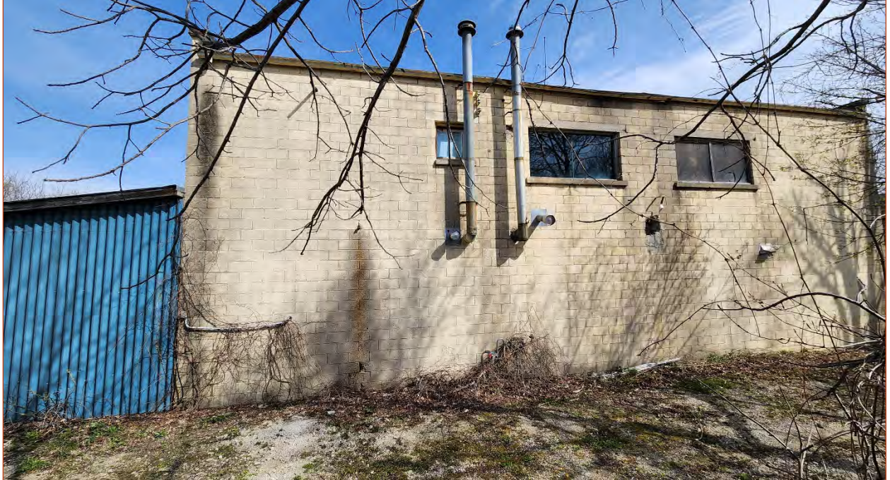
Image 17. View north of the south elevation
