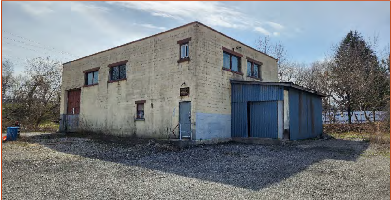
Image 15. View southeast of the north and west elevations
