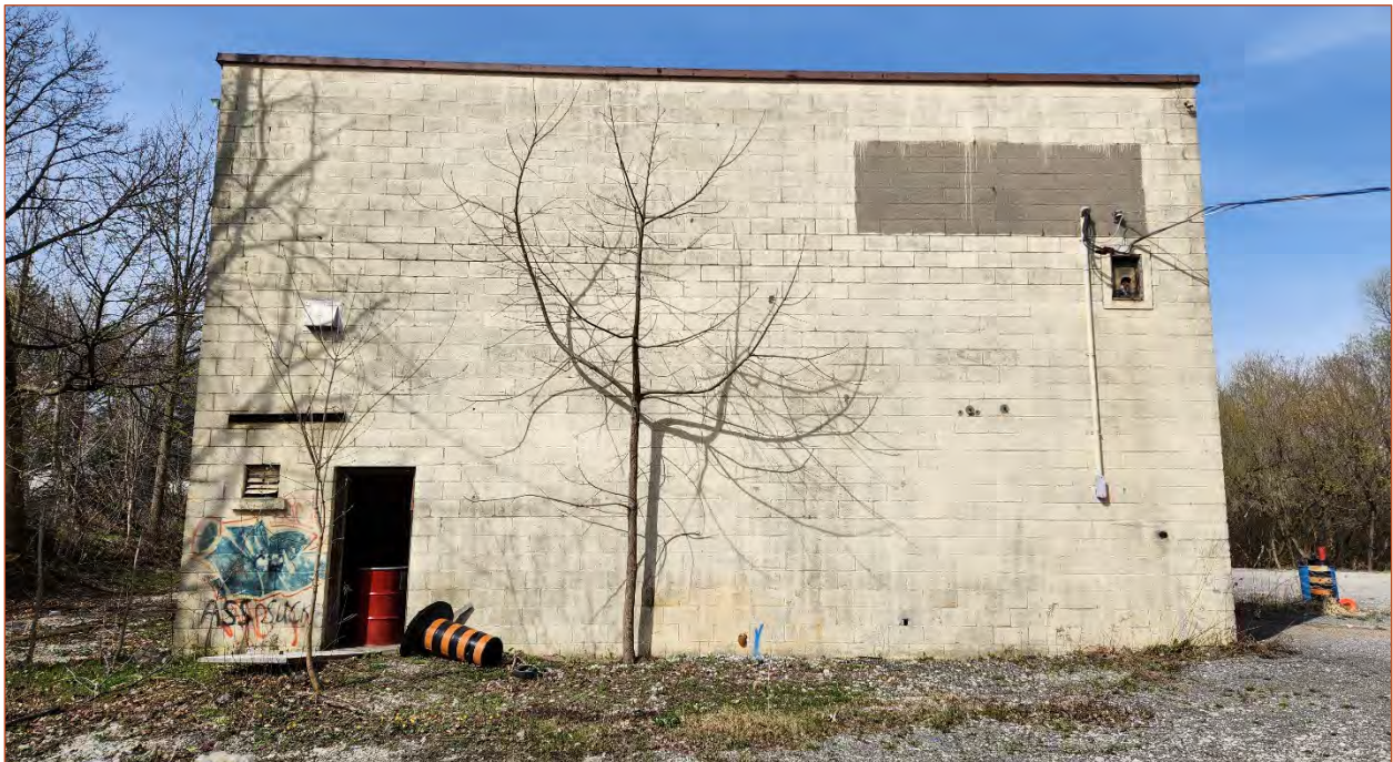
Image 16. View west of the east elevation
