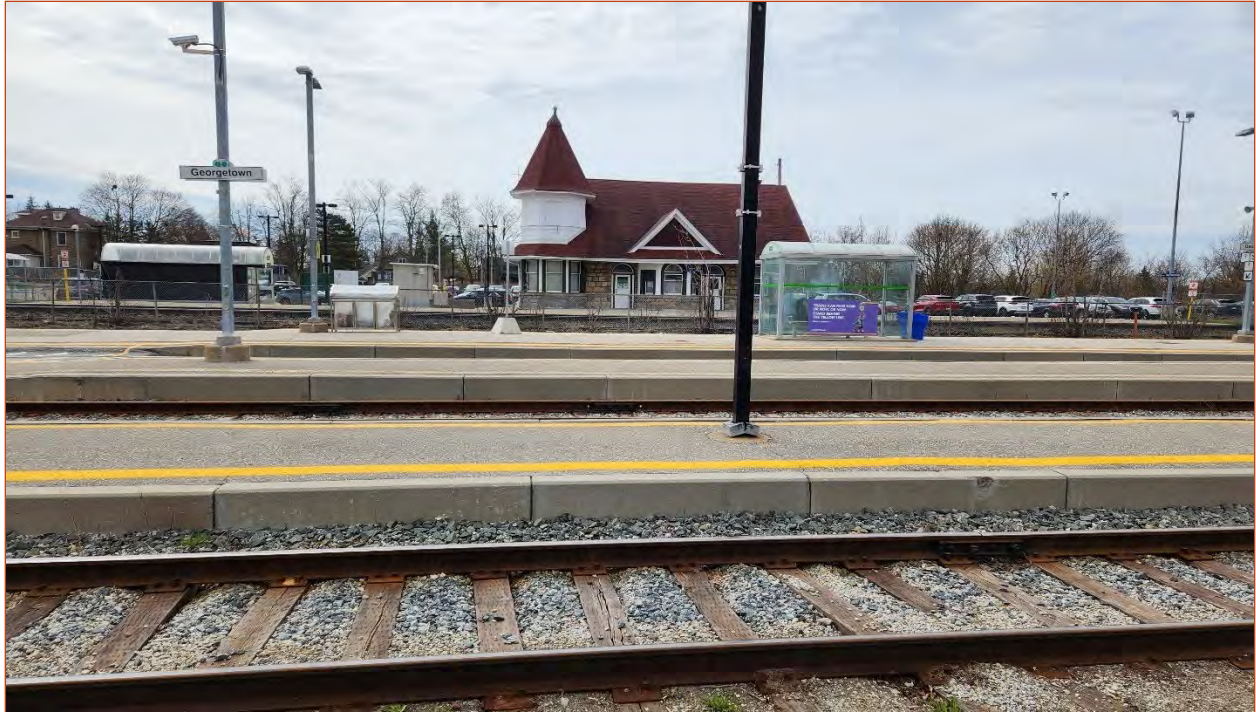
Image 10. View south of Georgetown GO Station building and tracks
