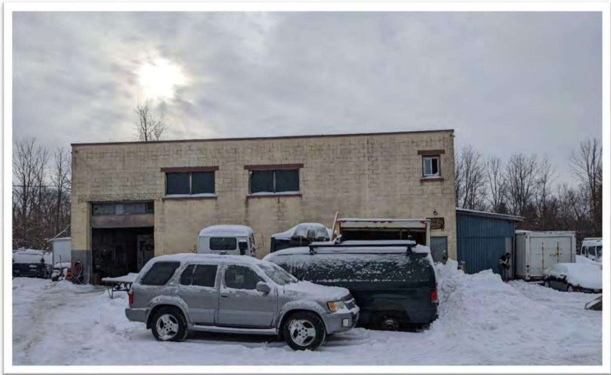
Photo 1: The Site exterior, facing south, front of the building.
