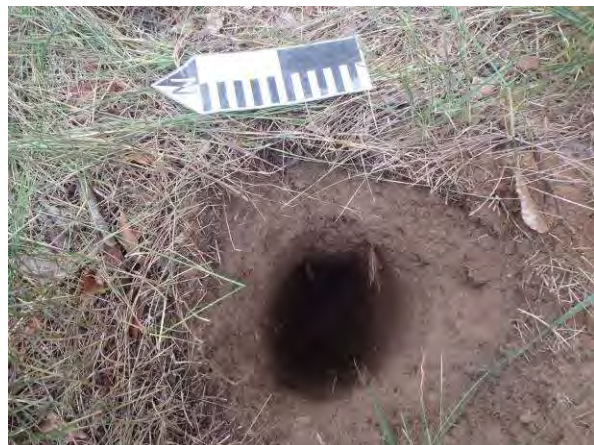
Plate 18: View of test pit with disturbed soil profile. Note test pit contained a laid topsoil layer, rocky fill, and gravel fill over subsoil.
