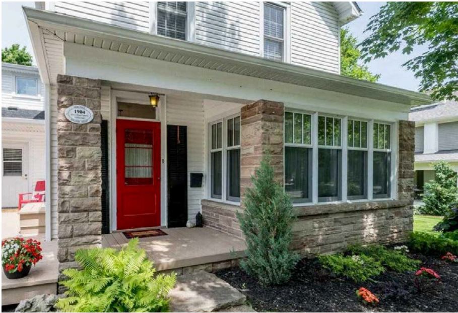
II. Before and after the restoration, as seen standing on Edith Street looking East toward 36 Edith Street, showing corbel, fretwork, brackets, posts, ceiling, door, and shutter details.
