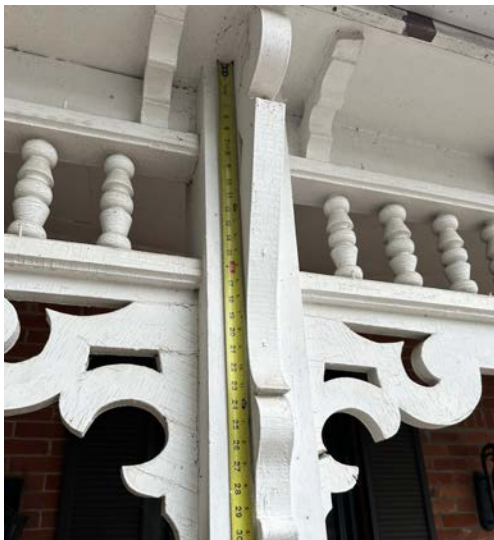
Top Left: corbels created using measurements found in original paint marks, using old-growth lumber from the property
