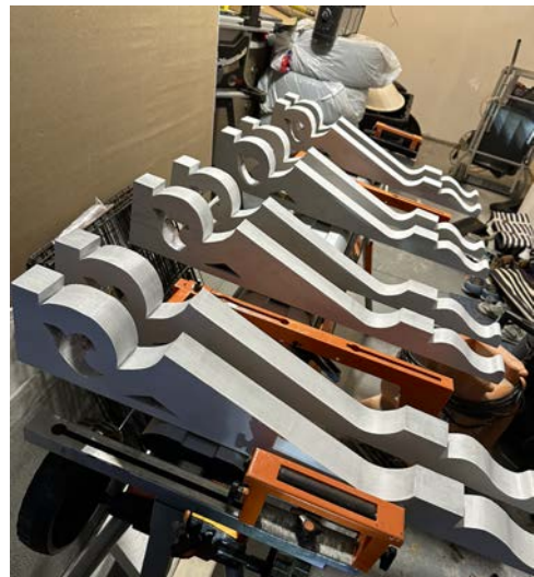
Top Left: corbels created using measurements found in original paint marks, using old-growth lumber from the property
