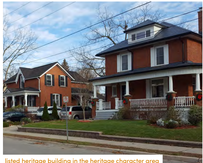
listed heritage building in the heritage character area
