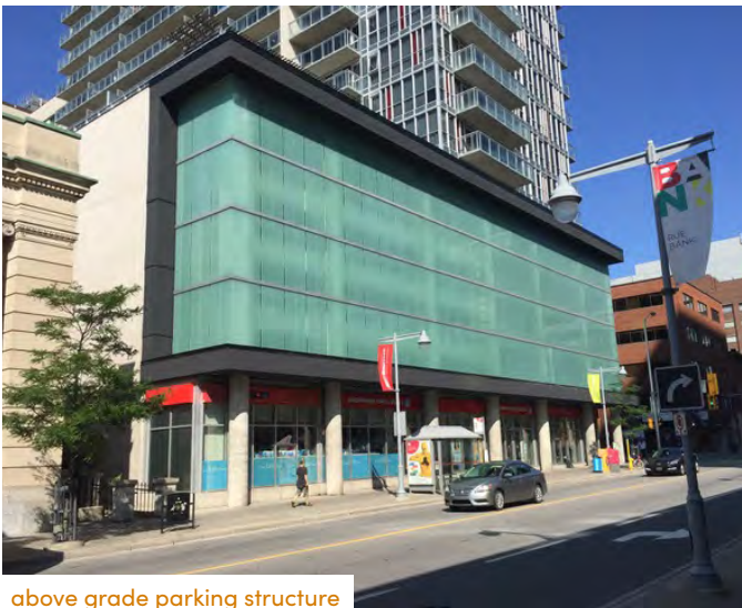
above grade parking structure
